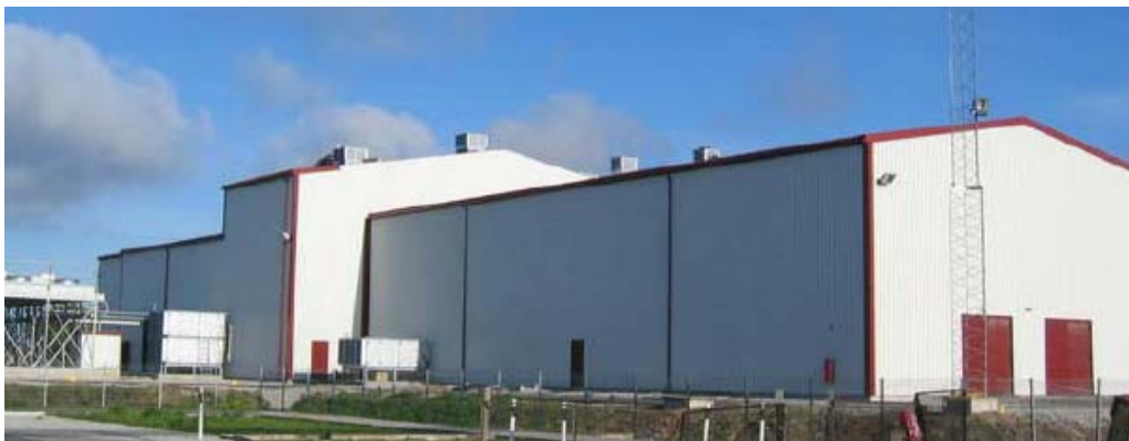
Figure 4-19 \pm 150 kV / 350 MW voltage source HVDC converter station at Harku, the Estonian terminal of the Estlink interconnector (source: [Ronström 2007])
