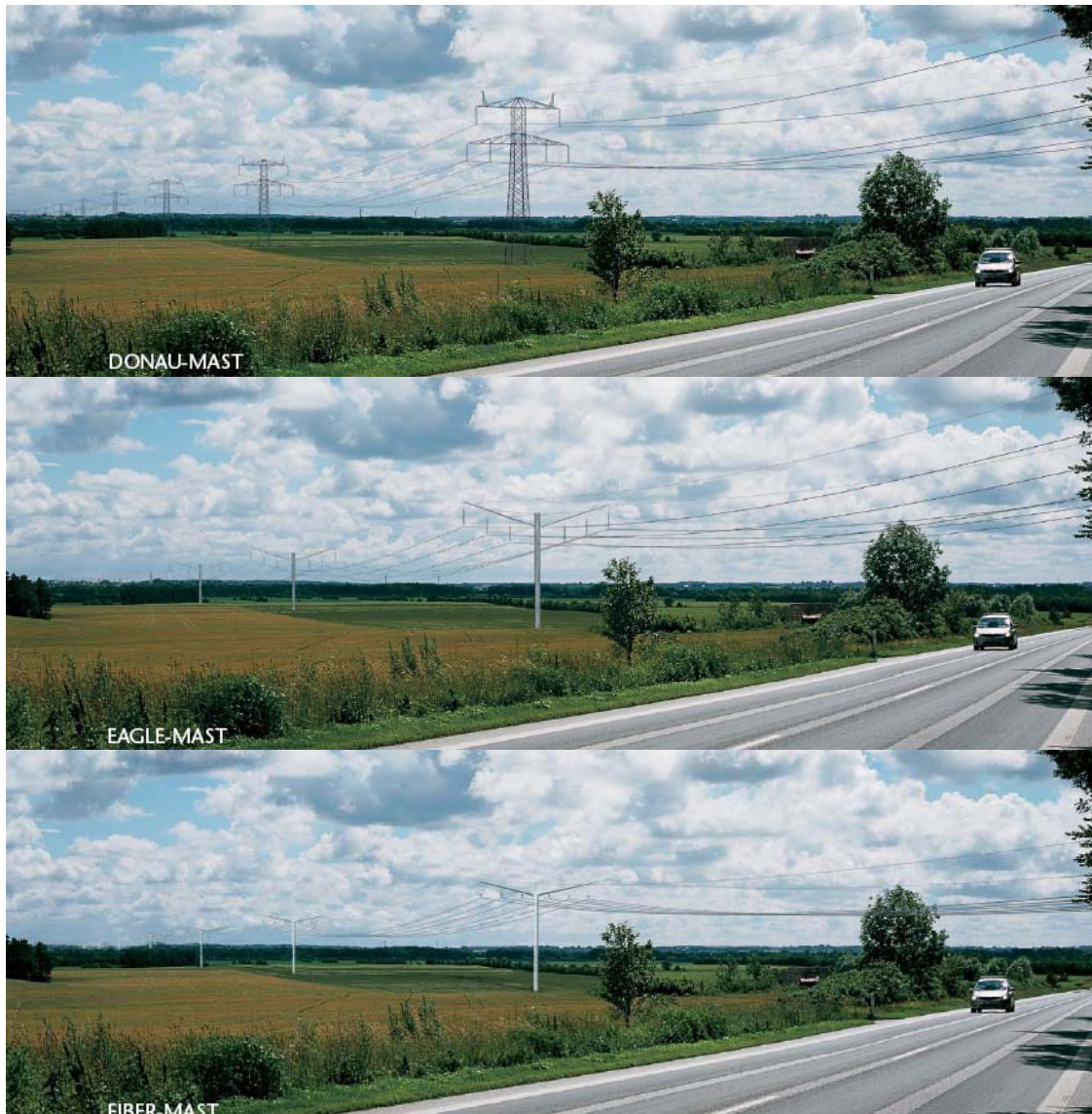
Figure 4-5 Conventional design (Donau-Mast) and new tower designs for improved visual impact [Energienet.dk]
