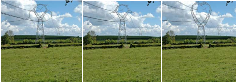
Figure 4-4 Tower Designs published by EirGrid, IVI (left), VVV (middle) and inverted delta (right) [EirGrid Web]
