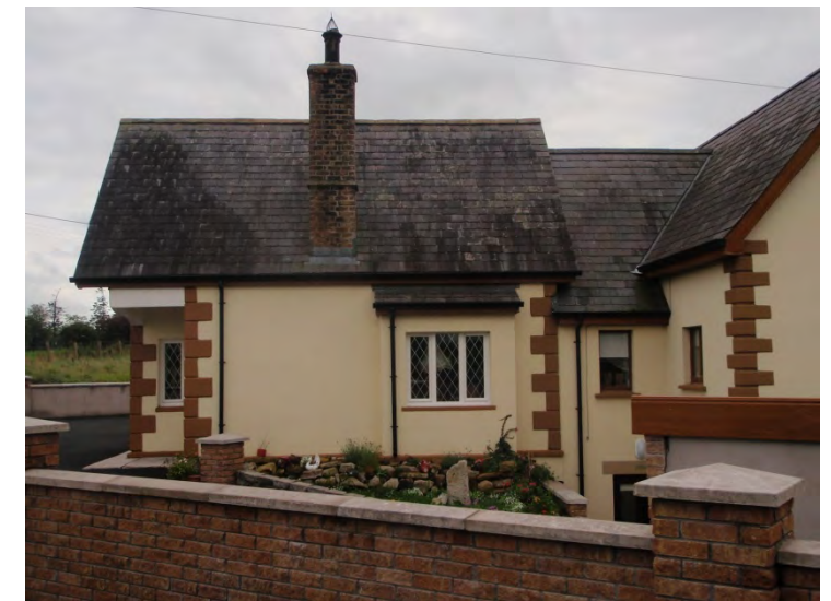
PHOTO 2 Original lodge to left with 2004 extensions to right
