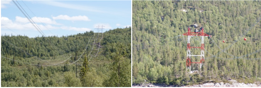
Traditional lattice steel tower painted in different colours in Norway.
