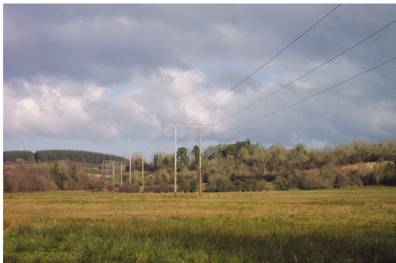
A typical 110kV overhead line
