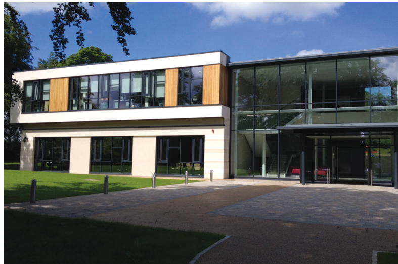
SONI Ltd Headquarters, Castlereagh House, Belfast
